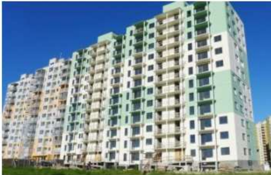
RESIDENTIAL BUILDING SMILGOS
