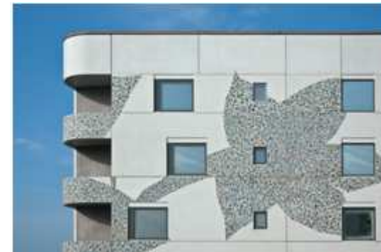
Flooranaukio Residence, Finland
