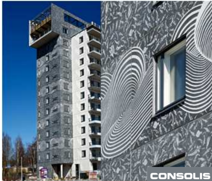
Graphic Concrete Facade, Finland, Iconic Award 2014
