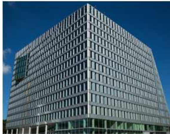
The Edge, World's most sustainable office building, Netherlands
