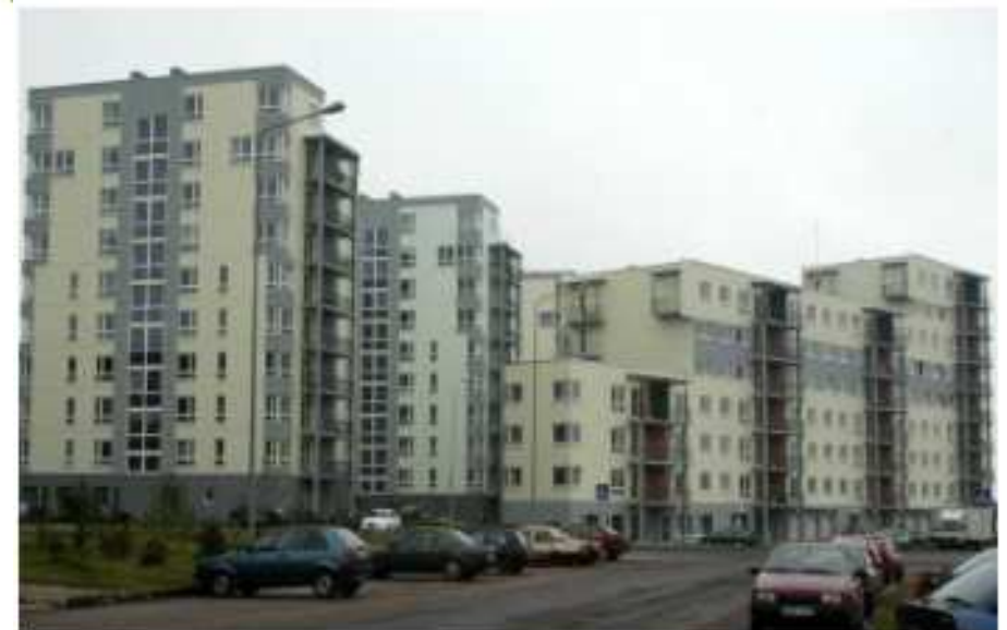
RESIDENTIAL BUILDINGS IN PILAITĖ (2)
