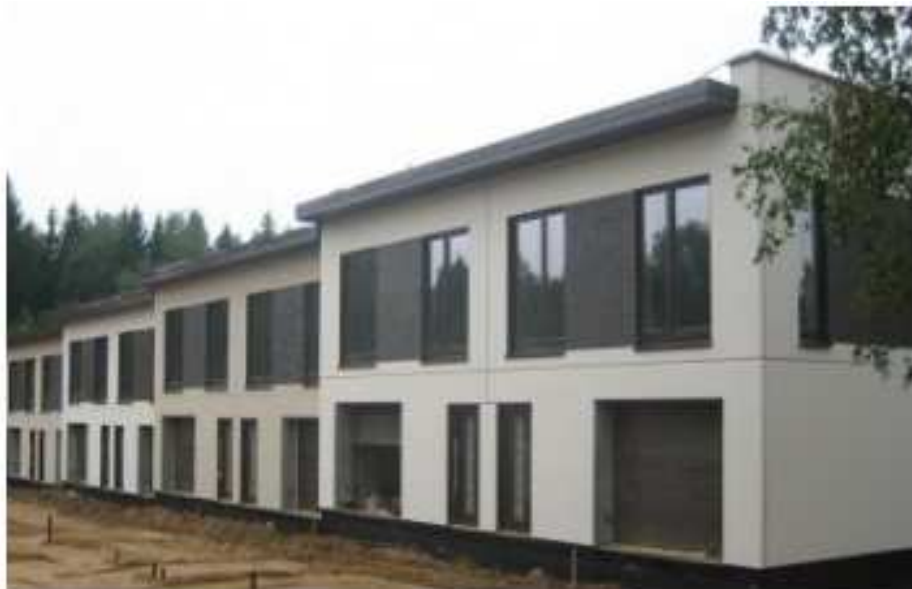
RESIDENTIAL BUILDINGS FROM LARGE-PANEL SLABS
