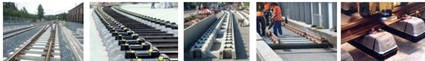
Bearers, Shallow depth twin block sleepers, Ladder track, Mono block sleepers, Twin block sleepers
