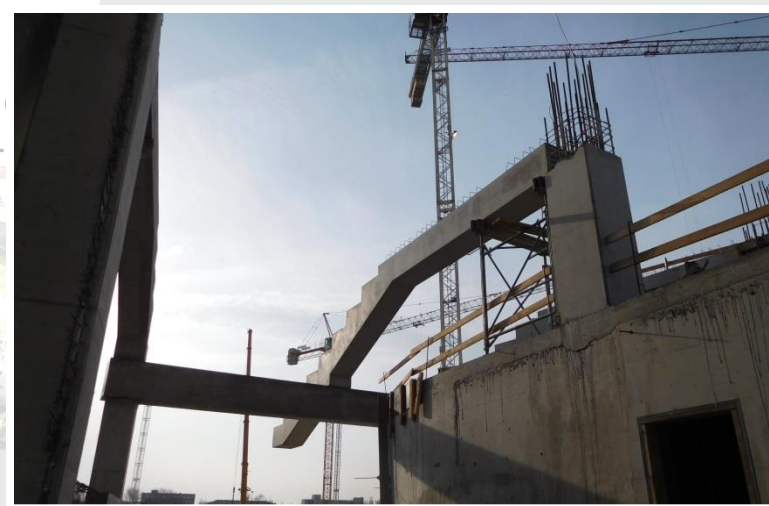
Case in site joints
