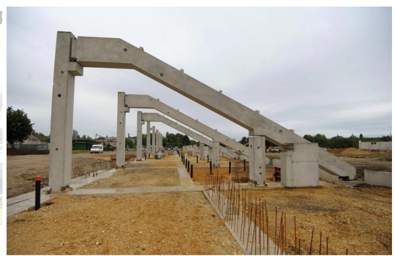
Case in steel structure
