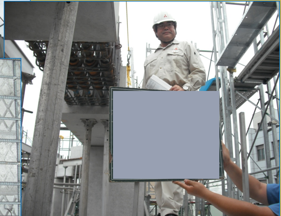
Inspection after grouting
