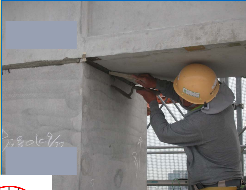
Column/column gap sealing
