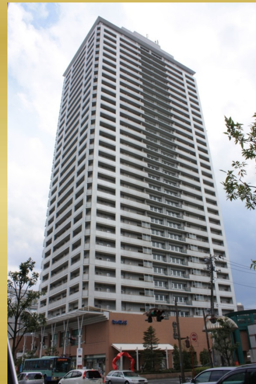
Moment frame structure building
