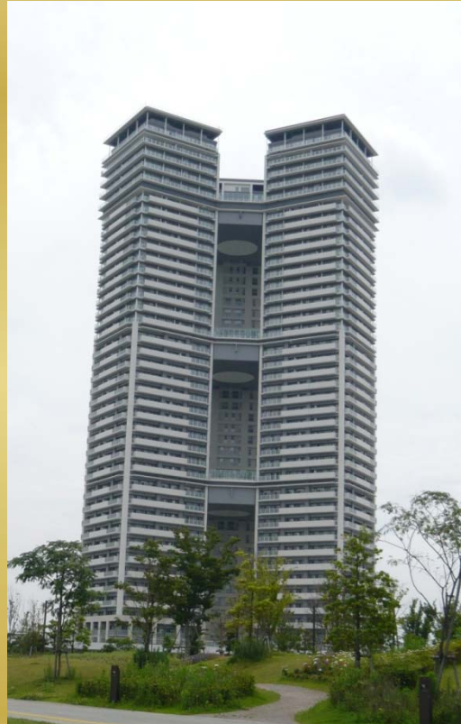
High rise building 42 stories, Fukuoka
