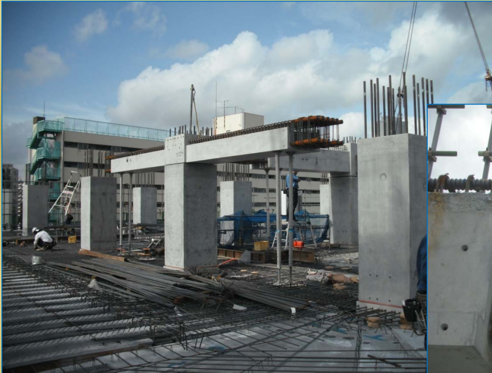
precast beam installation
