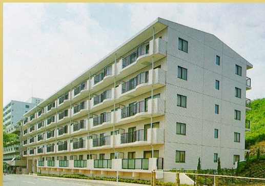
Wall structure building
