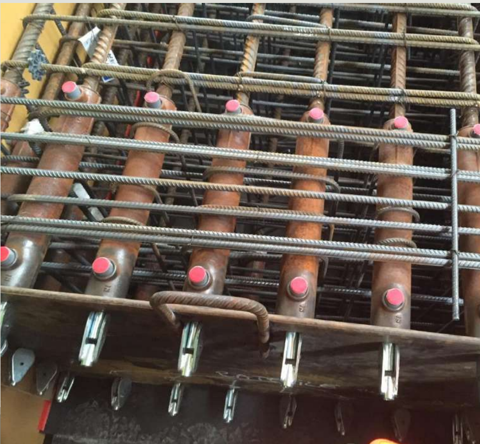
SPLICE SLEEVES INSIDE COLUMNS
